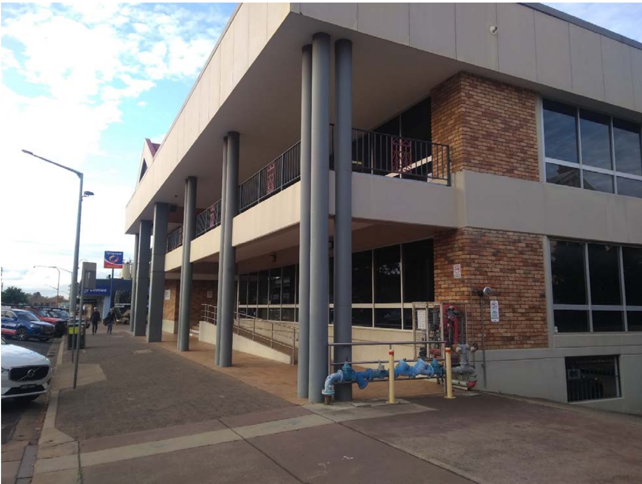
Looking north east toward the two storey office building located within 130 Brisbane Street. The building has two levels of office space and a single level basement car park with footprint equivalent to the overlying building. The basement car park is accessed by a ramped driveway on the southern side of the building.
