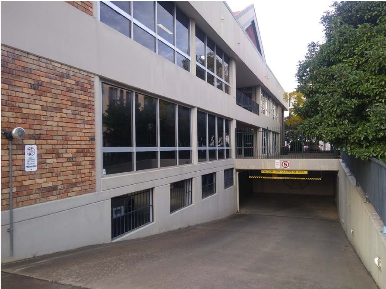
Looking north east toward the two storey office building located within 130 Brisbane Street. The building has two levels of office space and a single level basement car park with footprint equivalent to the overlying building. The basement car park is accessed by a ramped driveway on the southern side of the building.
